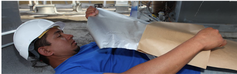
Peel back the width of your lap by a few inches, keeping the material as straight as possible as you begin installing.
