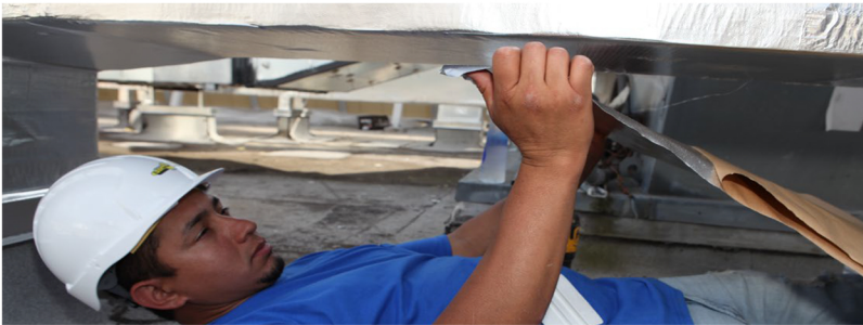
Use the provided squeegee to rub down the lap as you proceed. Pull the paper back as you come across the bottom of the duct work, smoothing out the material as you apply.
